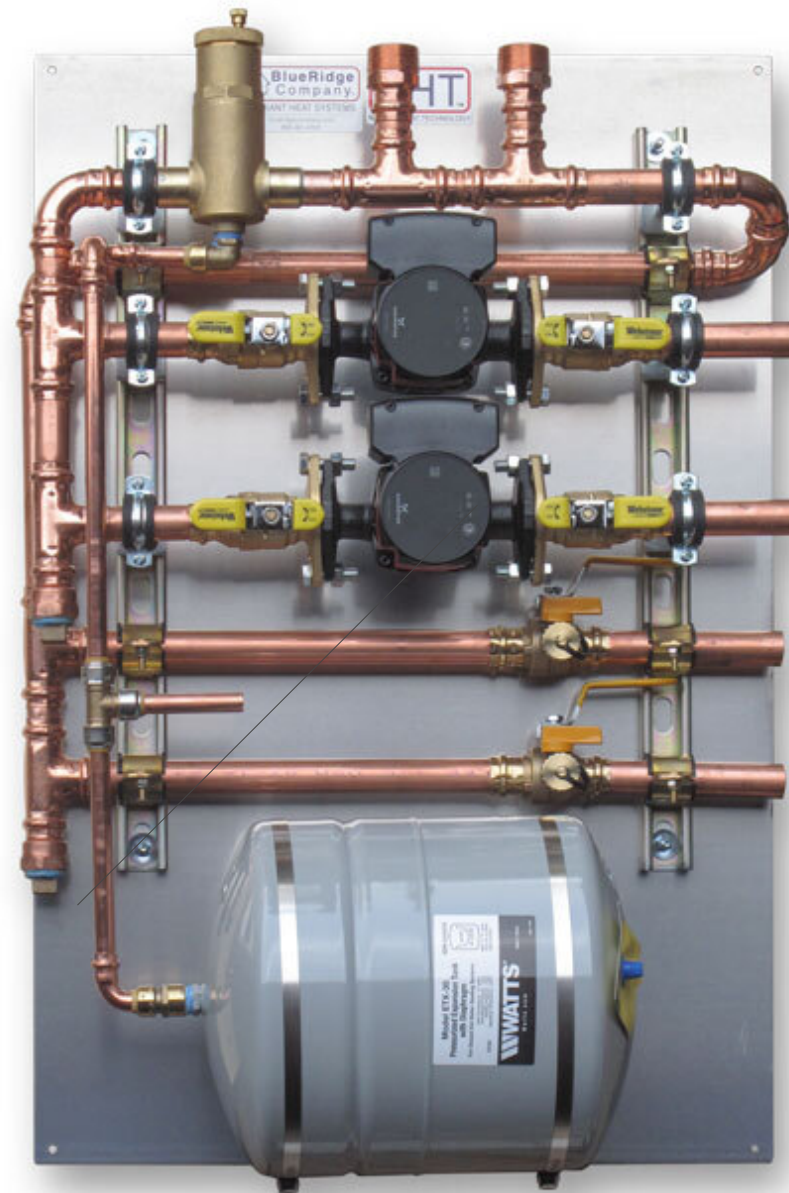
BlueRidge Company's RHT Prefabricated 2-Zone Column Pump Panel.
